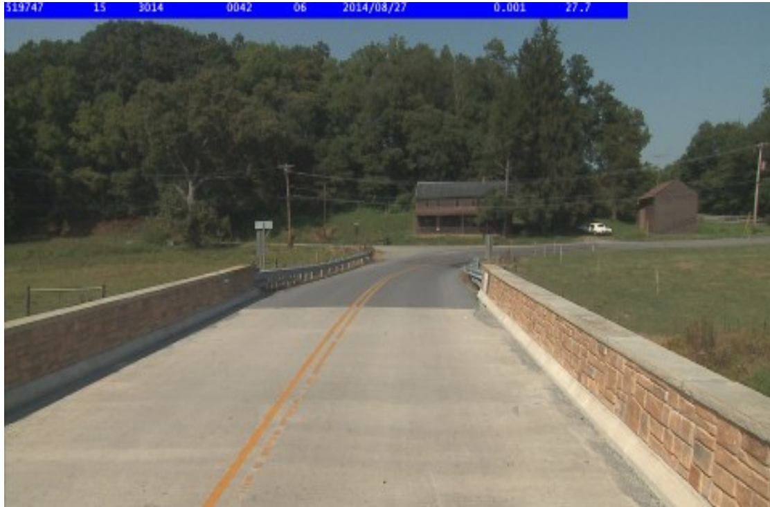
Photograph 1: Looking east toward the intersection of S.R. 3014 (Lees Bridge Road) and Sand Hill Road, West Nottingham Township, Chester County. Consulting parties requested a design similar to the Lees Bridge Road bridge for the S.R. 2002 Reynolds Run replacement bridge. (Photograph: PennDOT Videolog 2014)
